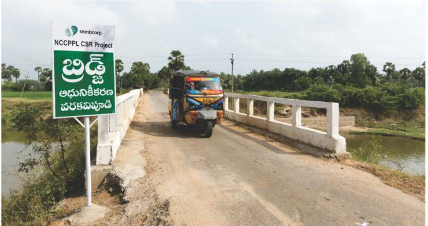
Improved transport access after renovation of bridge at Varakavipudi
