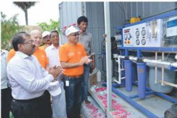
Inauguration of RO plant at Nelaturu BC&ST colony with Joint Collector
