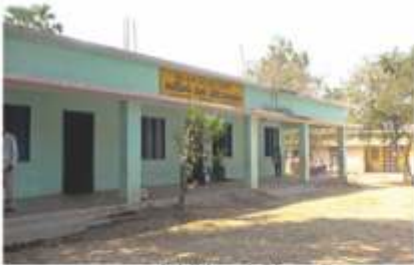
Additional Class Rooms in Musunurivarpalem
